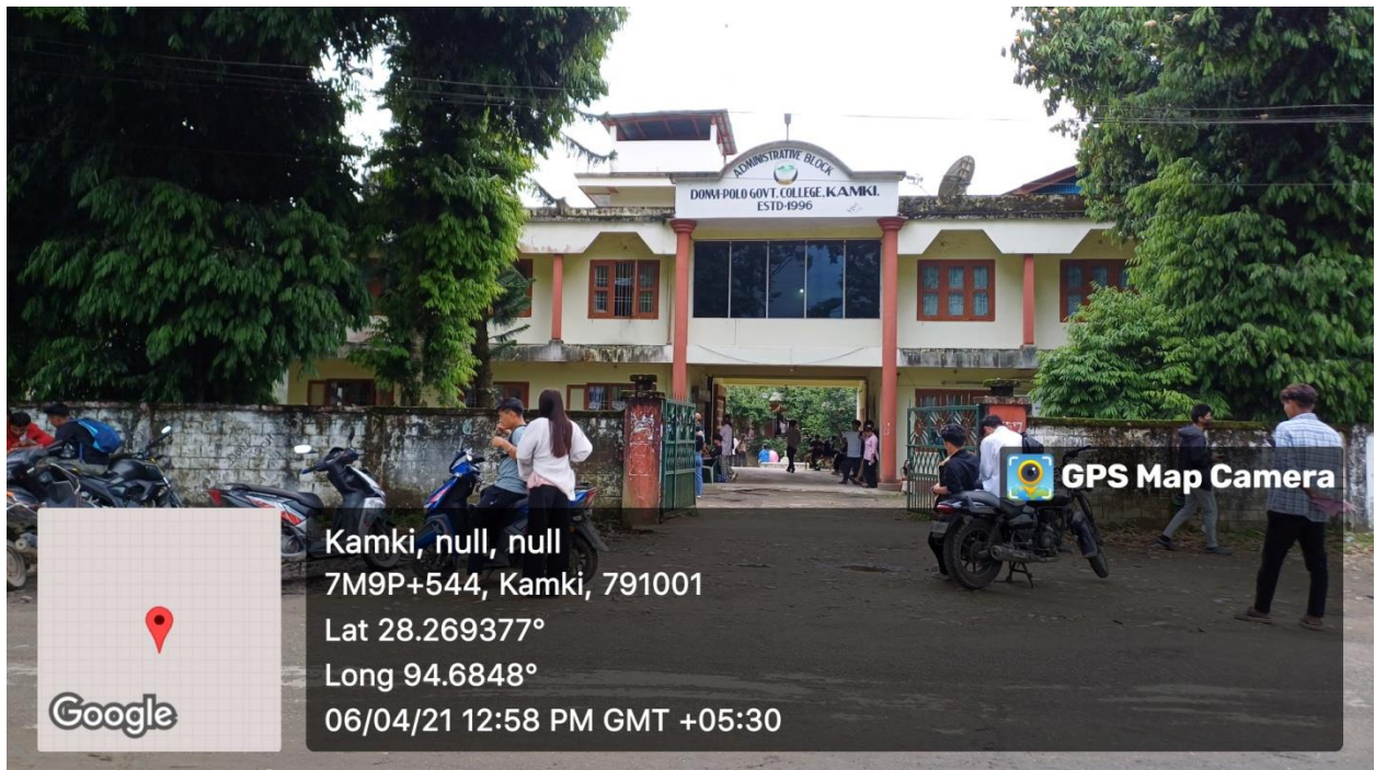
(Front of Administrative building)
