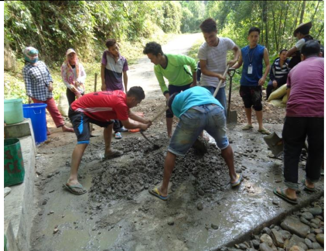
Mixing of Concrete Cement for Road Repairing
